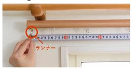
The width is measured from the center of the fixed runner.
